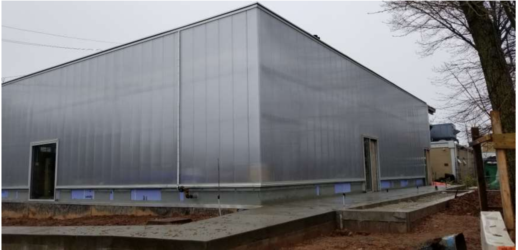
Exterior View of side ramp
